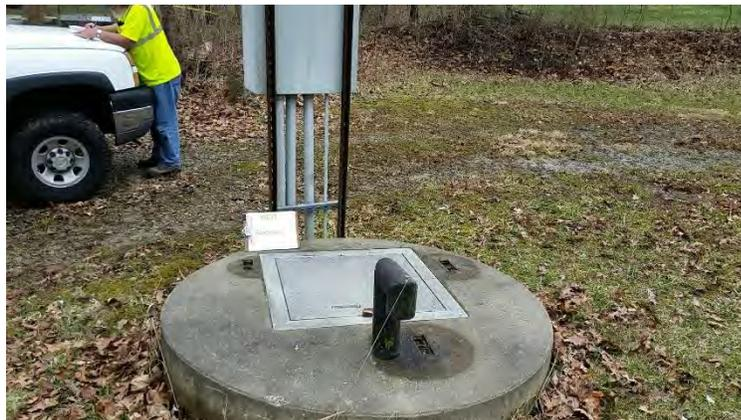
**Daycare** – Daycare is a duplex submersible pump station with a firm capacity of 100 GPM. The control panel is newer, and there is a broken private service line. This pump station is nearing capacity and should be evaluated as the facilities that it serves continue to grow. There is no permanent surrounding fence for protection. This pump station is shown in Figure 5-21 below.
