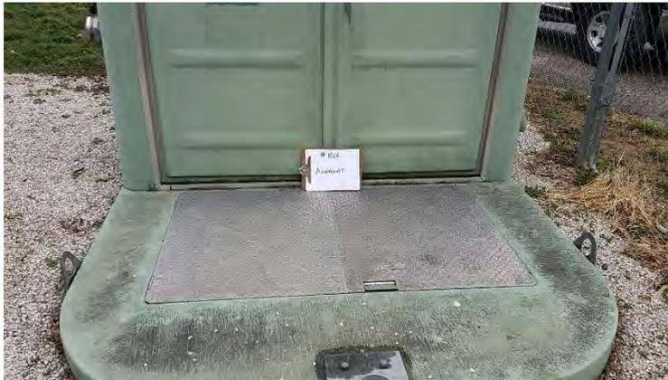
**Diversified Metal** – Diversified Metal is a duplex submersible pump station with a firm capacity of 57 GPM. This pump station only serves one (1) building, and City staff feels responsibility for maintenance should fall to Owner instead of City. This pump station will be decommissioned with the construction of the South Booster Pump Station and associated gravity piping. This pump station is shown in Figure 5-24 below.
