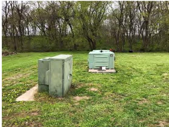
**Rock Creek** – Rock Creek is a duplex above-ground self-priming pump station. The firm capacity of the pump station is 175 GPM. It is of newer construction and still contains its original components. The area it serves is not fully built out and the pump station has not reached its capacity. There is no fence for protection. This pump station is shown in Figure 5-4 below.
