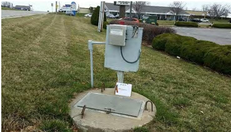
**Platte Valley** – Platte Valley is a duplex submersible pump station with a firm capacity of 100 GPM. The pumps were replaced in 2006 and the control panel was replaced in 2013. This pump station will be decommissioned with the construction of the South Booster Pump Station and associated gravity piping. This pump station is shown in Figure 5-26 below.
