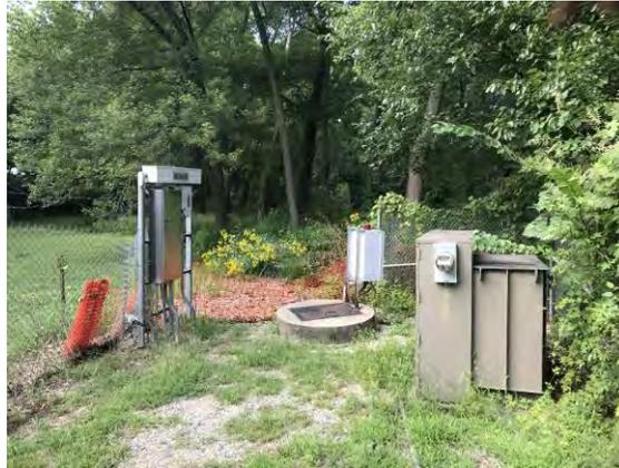
**Cub Cadet** – Cub Cadet is a duplex submersible pump station. It serves a small area collecting flow from three bathrooms. The City has replaced the pumps and the controls for this pump station. This pump station is shown in Figure 5-13 below.
