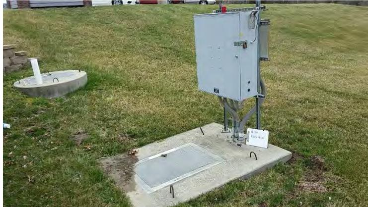
**Hills of Shannon** – Hills of Shannon is a duplex above-ground self-priming pump station with a firm capacity of 300 GPM. This pump station will be decommissioned with the construction of the South Booster Pump Station located on 144<sup>th</sup> Street. This pump station is shown in Figure 5-27 below.
