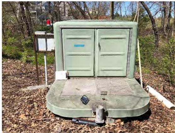
**Strawberry Hill** – Strawberry Hill is a duplex above-ground self-priming pump station built in approximately 2005. There is no fence for protection and the gravel on the access road stops short of the pump station. This pump station is shown in Figure 5-18 below.
