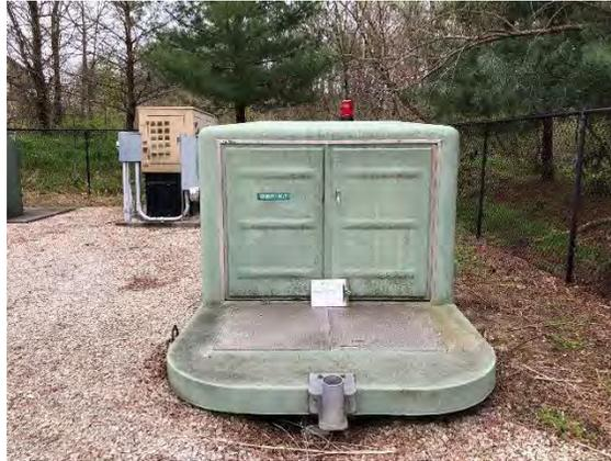
**Greyhawke 2** – Greyhawke 2 is a duplex submersible pump station with a firm capacity of 90 GPM. The pumps are original. The transducers that were installed caused issues with the controls and have been replaced with floats. The City has replaced the rails and piping at this pump station. This pump station is lacking an access road altogether and one should be constructed. This pump station is shown in Figure 5-7 below.
