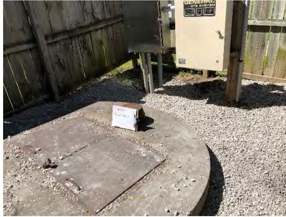
**Stone Creek Villas** – Stone Creek Villas is a duplex submersible pump station with a firm capacity of 30 GPM. This pump station is located directly next to private property, and there is no room for a fence. The pumps are newer, but there are some electrical wiring issues including a seal pad contact that shows inaccurate readings on Mission. The access road to this pump station is not paved, and should be upgraded. This pump station is shown in Figure 5-15 below.
