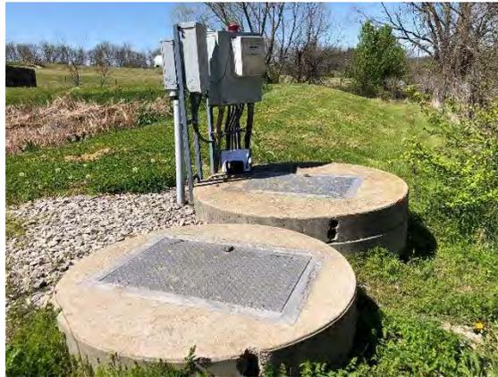
**Cedar Lakes 1** – Cedar Lakes 1 is a duplex submersible pump station with a firm capacity of 275 GPM. The pumps and control panel are newer. This pump station is located in a private park. There is no fence for protection and no direct access road. If needed, a vehicle can access the pump station by driving through the park, but this is not preferable. This pump station is shown in Figure 5-16 below.
