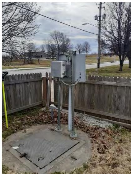
**Stone Bridge** – Stone Bridge is a duplex submersible pump station. This pump station pumps to the Daycare Pump Station. The control panel has been upgraded, but the pump station is lacking a fence for protection. Grease is an ongoing issue with this pump station and requires regular maintenance from City staff. This pump station is shown in Figure 5-22 below.
