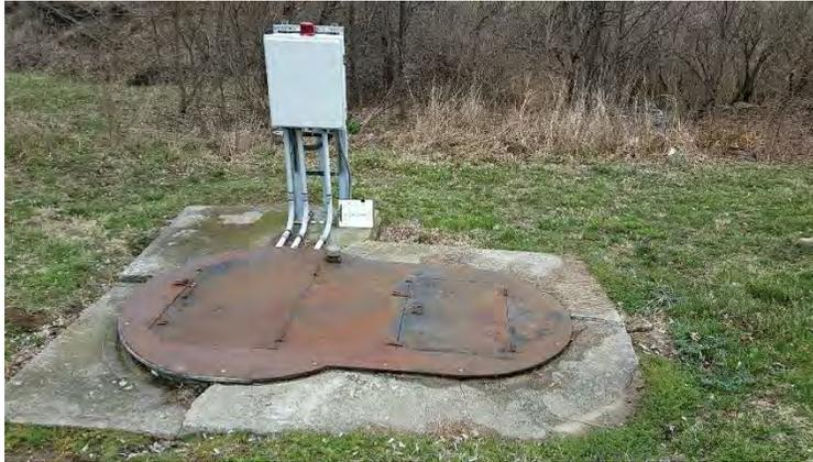
**Ashmont** – Ashmont is a duplex submersible pump station that was installed in approximately 2007. The pump station has a firm capacity of 100 GPM. Both pumps were replaced in 2018. The fence and paved access road are suitable for City staff. Grease is an ongoing issue with this pump station and requires regular maintenance from City staff. This pump station is shown in Figure 5-23 below.
