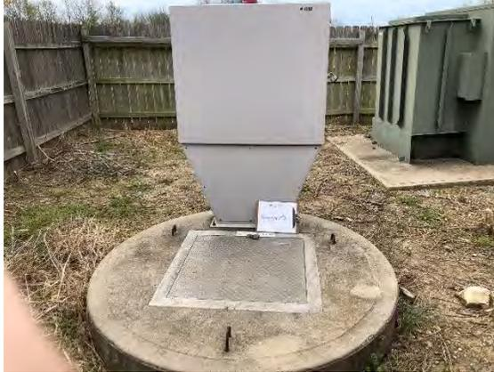
**Big Harborview** – Big Harborview is a duplex above-ground self-priming pump station with a firm capacity of 375 GPM. This pump station serves the Clay County Park restrooms and the beach on the north side of Smithville Lake. There is a large detention basin with sufficient holding capacity. The fencing should be upgraded and access road has previously been rebuilt. This pump station is shown in Figure 5-11 below.
