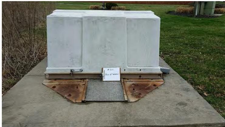
**Gerber Collision** – Gerber Collision is a duplex submersible pump station with a firm capacity of 30 GPM. It serves two building and has few issues. This pump station is shown in Figure 5-28 below.
