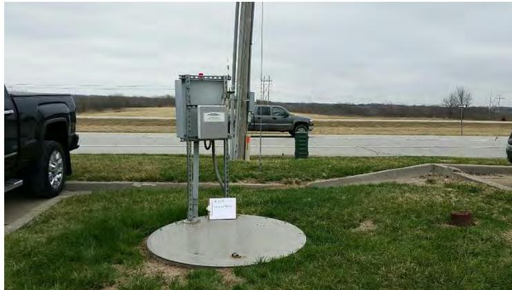
**Woods Court** – Woods Court is a duplex submersible pump station with a firm capacity of 105 GPM. It has an upgraded control panel and a large wetwell. There are occasional issues with this pump station on the weekends, but it rarely goes high. This pump station is shown in Figure 5-29 below.
